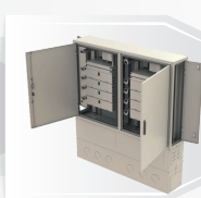
Street Type Twin Cabinet FDF-ODC-2-X
