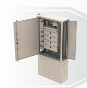
Street Type Cabinet FDF-ODC-2
